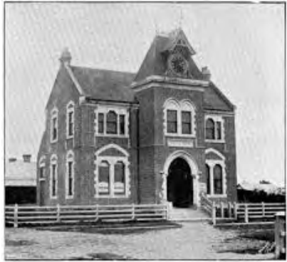
ASHBURTON BOROUGH COUNCIL CHAMBERS AND TOWN LIBRARY
